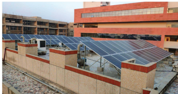
RENEWABLE ENERGY GENERATION THROUGH INSTALLATION OF 200KW SOLAR PANELS
