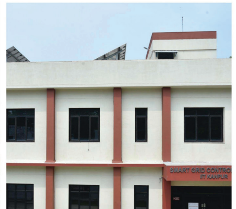
SMART GRID CONTROL CENTRE
