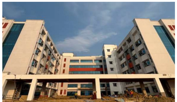
Latest view of the GSMST construction site
