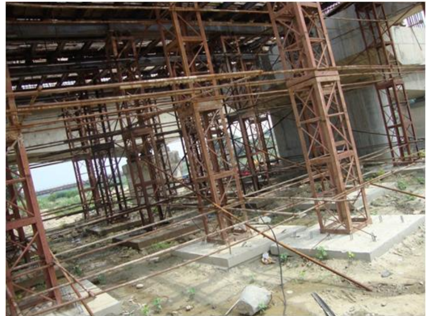
Another view of bridge formwork- Reinforcement is being used as bracing
