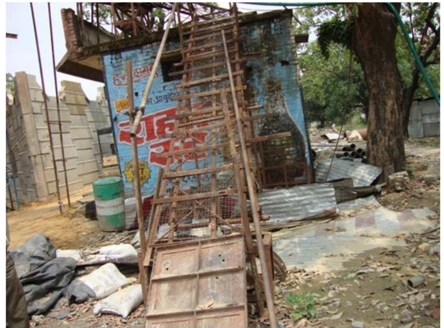
Another view of access to workplace
