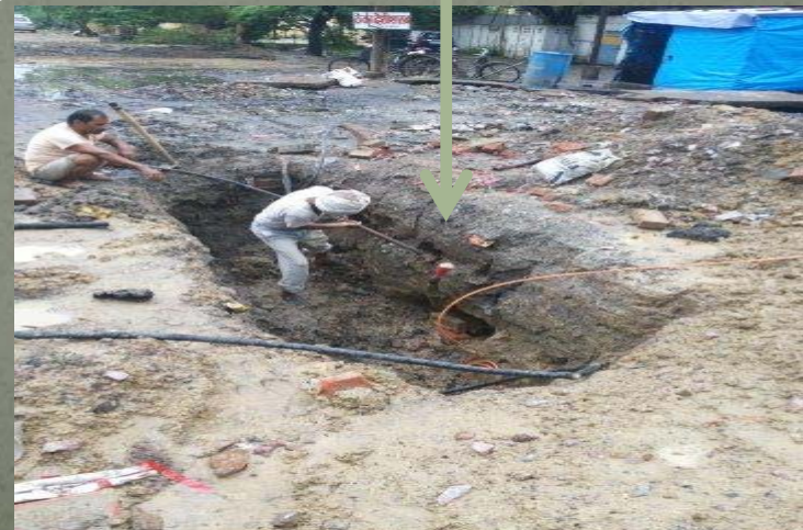
Gas Leakage Started here and got fire due to tea stall flame
