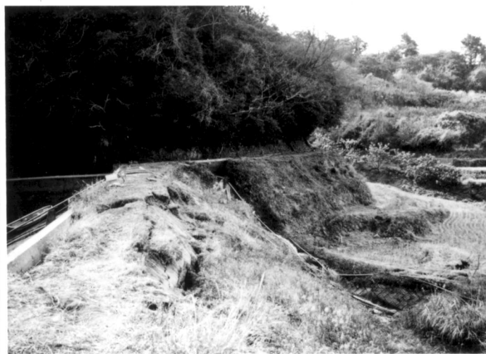
Fig. 12. Damage to Izuminaka Dam close to Nojima Fault
