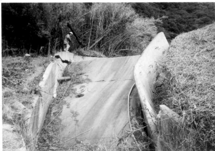
Fig. 11. Damage to the spillway on Mukumoto Dam close to Nojima Fault
