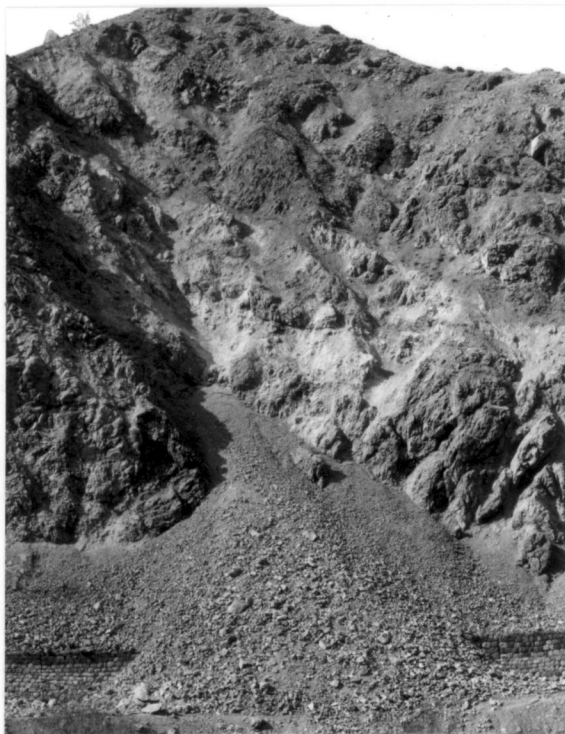
Photo 7 Rock slope failure near Tanyeri
