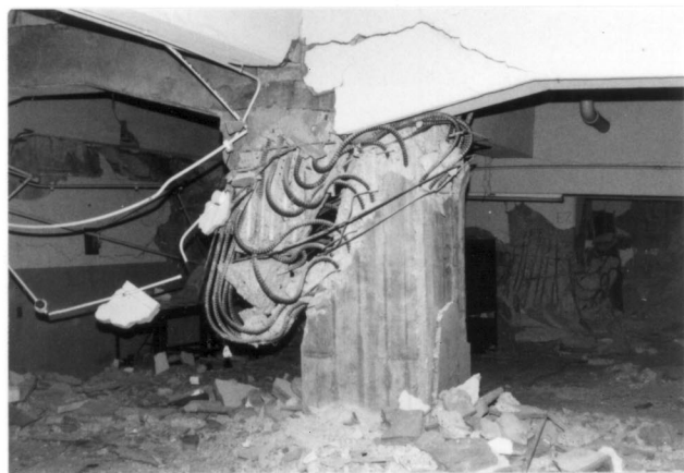
(a) shear failure of the first-story columns
