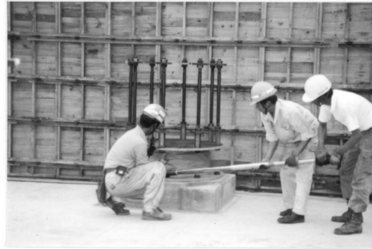
Fig. 5-2. Installing a laminated rubber bearing
