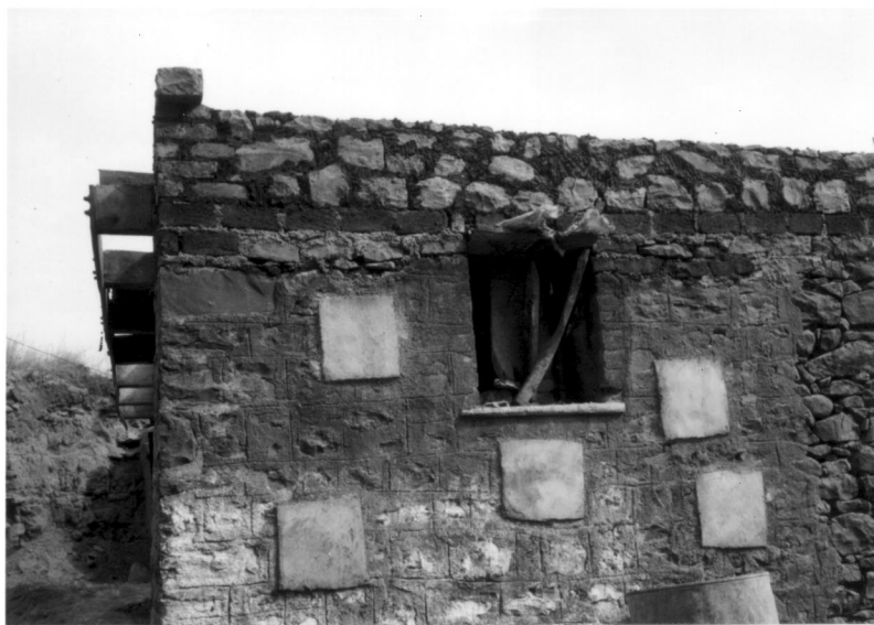
Fig. 4. A field application of retrofitting methodology showing ring beam installed at the eaves level including reconstruction of parapet walls, and through-stones installed in a stone wall (Kharosa village, Marathwada).
