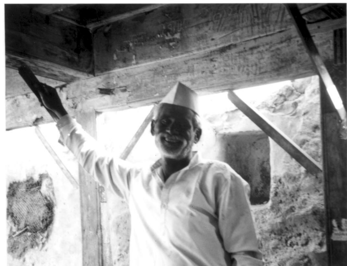
Fig. 5. Knee-bracing of a timber frame: a) Detail of a rolled steel angle bracing, and b) Field application in a rural house, Marathwada.
