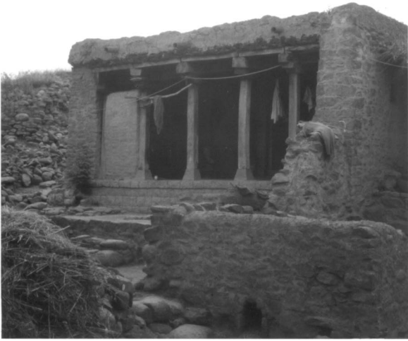
Fig. 1. A traditional stone masonry house with timber frame in a Marathwada village.
