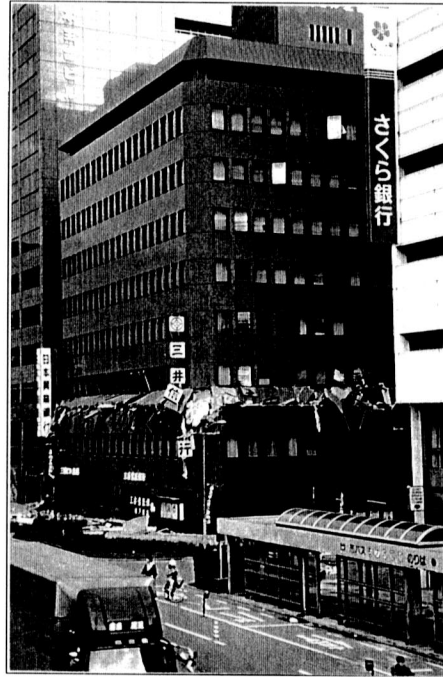
Photo 3 Damage to an intermediate floor collapse-type
