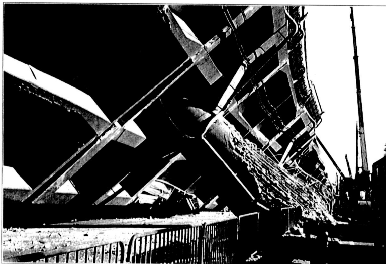
Photo 5 Collapse of pilz-type bridges
