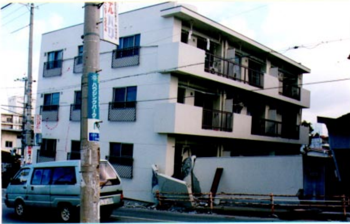
Fig. 5. Class D building with grade 5 damage.
