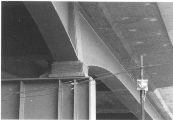
Photo-1 Pelham Bridge Rubber Bearing In 1994
