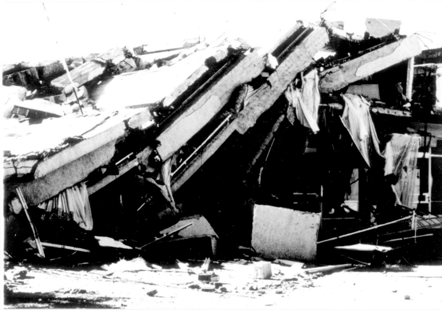
Fig. 4. Structural hazard : 1995 Dinar Earthquake
