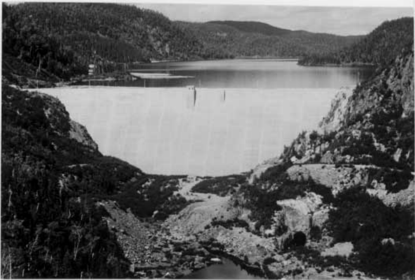
Fig. 1: Aerial view of Outardes 3 gravity dam with full reservoir
