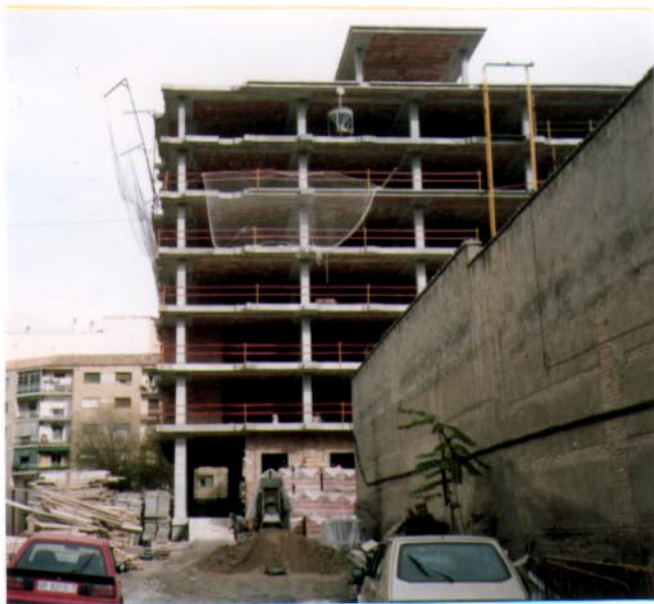
Photo. 2 Apartment building, Plaza de Toros (under construction in 1993)
