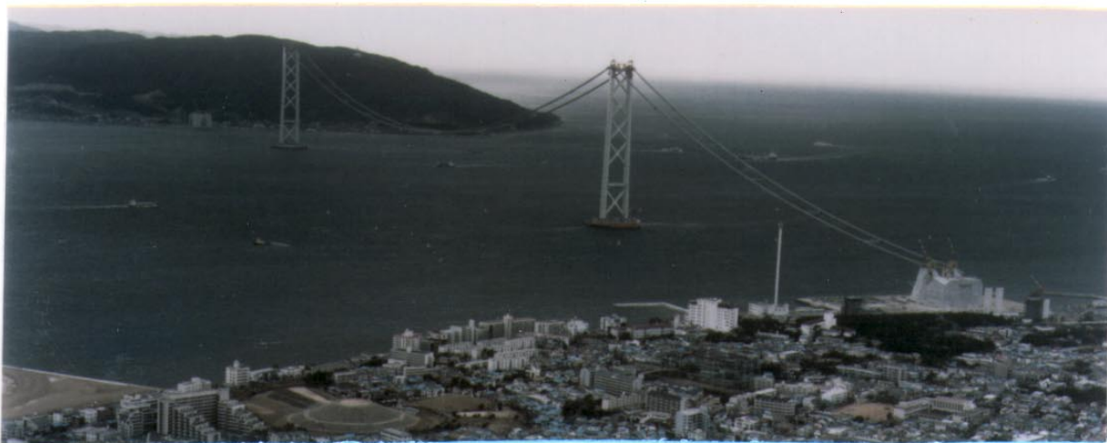
Photo 1 Construction work in progress at the Akashi Straits
