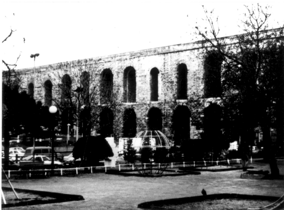
Fig. 1. A central view of Bozdogan (Valence) Aqueduct, Istanbul.
