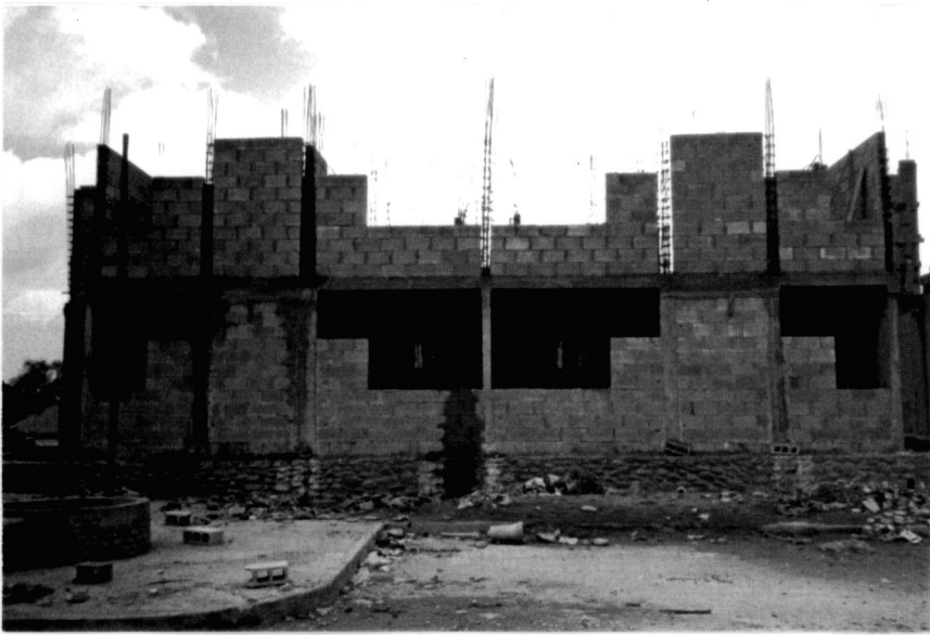
Fig. 1. Confined masonry walls using hollow concrete-block masonry units. (Las Losas Project under construction in Villahermosa, Mexico)
