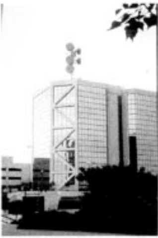
Fig. 1 Communication equipment on building
