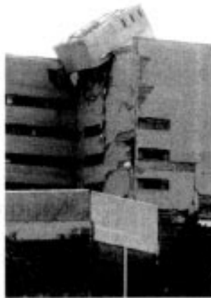
Fig. 5 Penthouse failure
