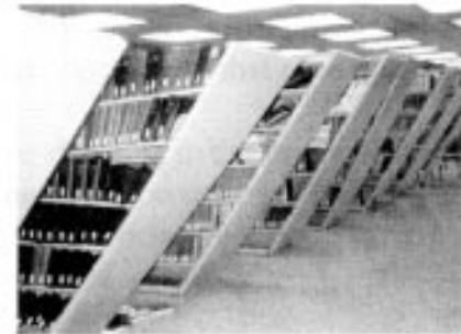
Fig. 9 Damaged bookshelves (After Taly, 1988)
