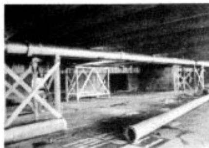
Fig. 8 Collapsed pipe in parking garage (After Rihal, 1990)
