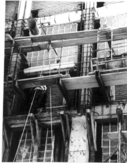
Fig.6 Seismic strengthening by jacking structural elements. Milling building in Costa Rica.
