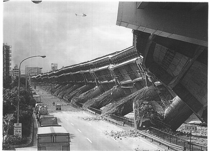
Photo 1 Collapse of Viaduct at Fukae, Kobe on Hanshin Expressway Route 3
