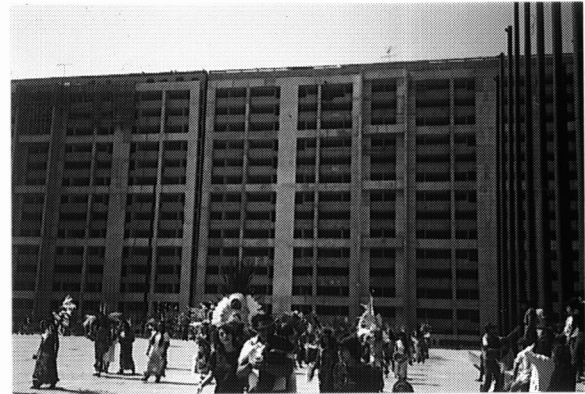
Photo 4 Concrete jacketing (after 1985 Mexico earthquake)
