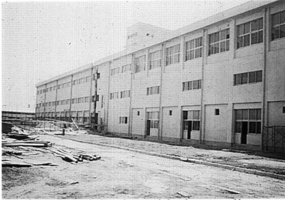
Photo 1 Strengthening with shear walls (after 1968 Tokachi-oki earthquake)
