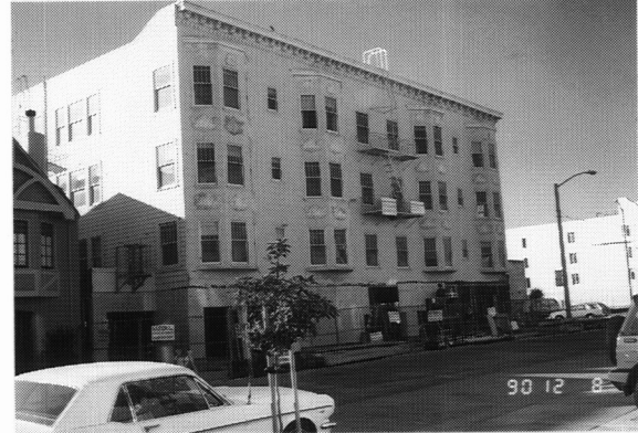
Photo 6 Rehabilitation with seismic isolation (after 1989 Loma Prieta earthquake)
