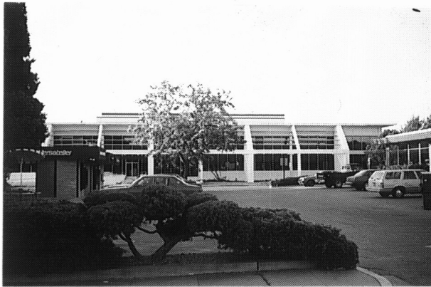
Photo 3 Strengthening with buttresses (after 1980 Livermore earthquake)
