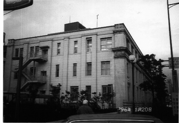
Photo 9 An old building in Kobe rehabilitated ten months before the earthquake of 1995 (no damage)
