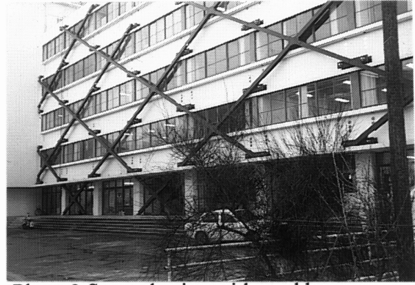
Photo 2 Strengthening with steel braces (after 1978 Miyagiken-oki earthquake)
