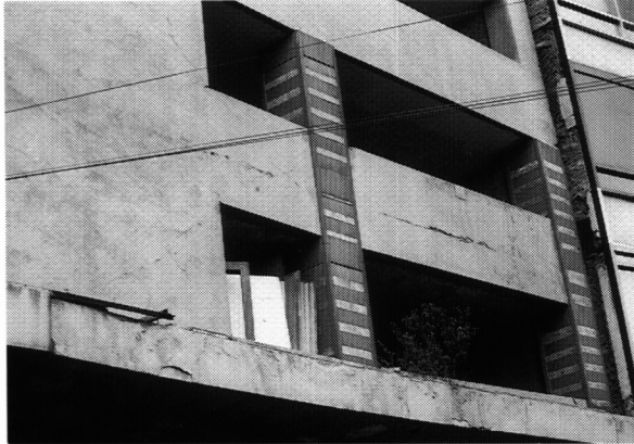
Photo 5 Steel jacketing (after 1985 Mexico earthquake)
