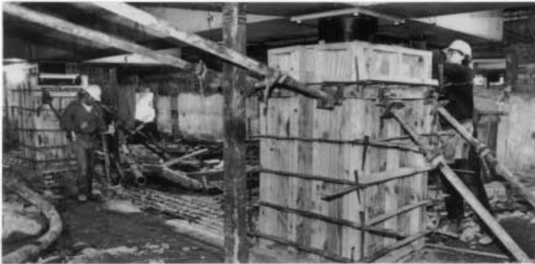
Figure 6 Lead-rubber bearings being retrofitted under New Zealand Parliament
