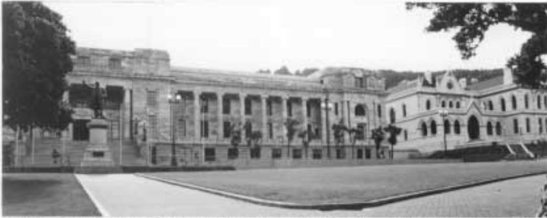
Figure 5 New Zealand Parliament and Assembly Library after retrofit with lead-rubber bearing isolators.
