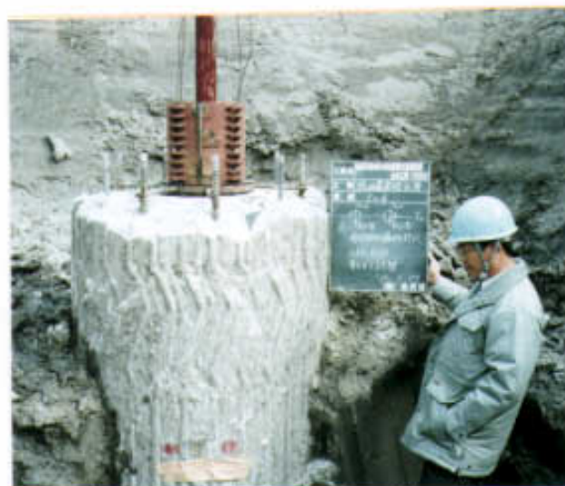
(b) Photo of Field Test Situation
