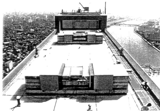
Fig.5. Scene of device installation
