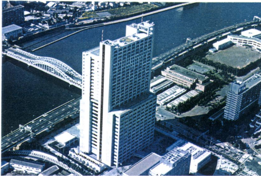
Fig.1. View of the entire of the building
