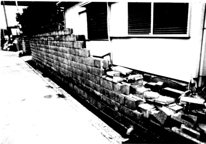
Fig. 11. Masonry wall without wall Re-bars.
