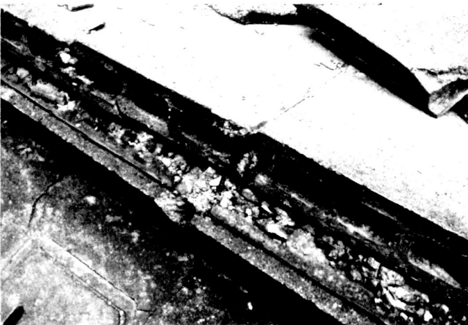
Fig. 13. Insufficient anchorage for vertical Re-bars.
