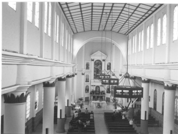
Photo 3. Interior view of the church toward the Presbytery
