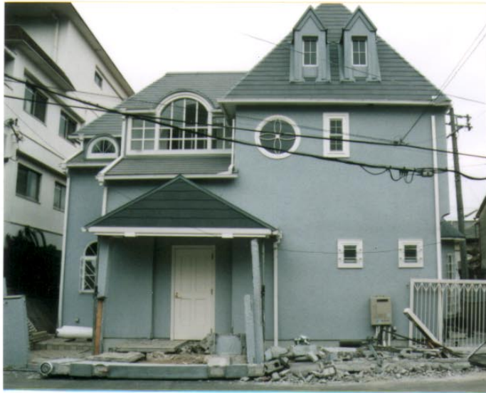
PICTURE 3 TWO-BY-FOUR CONSTRUCTION
