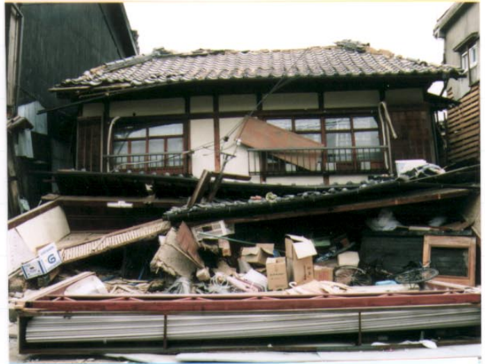
PICTURE 2 OLDER POST AND BEAM CONSTRUCTION
