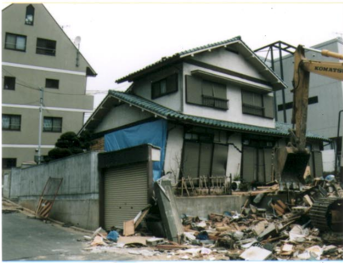
PICTURE 1 MODERN POST AND BEAM CONSTRUCTION
