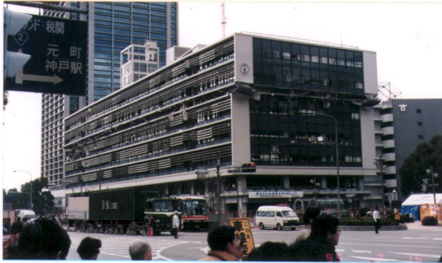
Photo.1. Complete collapse of mid-height story of a eight story building.
