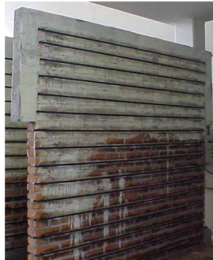
Fig. 3: Unreinforced masonry wall
