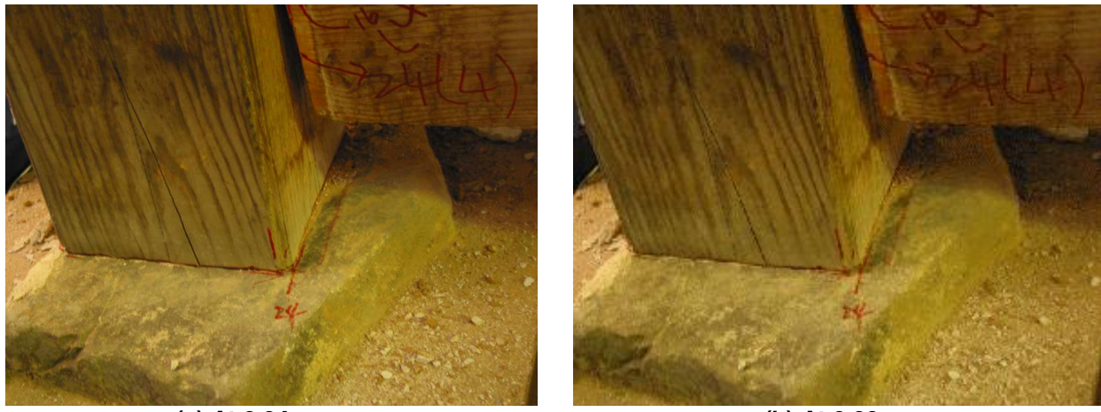
(a) At 0.24g (b) At 0.28g Figure 9. Close-up view of the movement of column base
