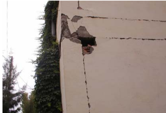
Photo 4.3: Masonry-structure interaction
