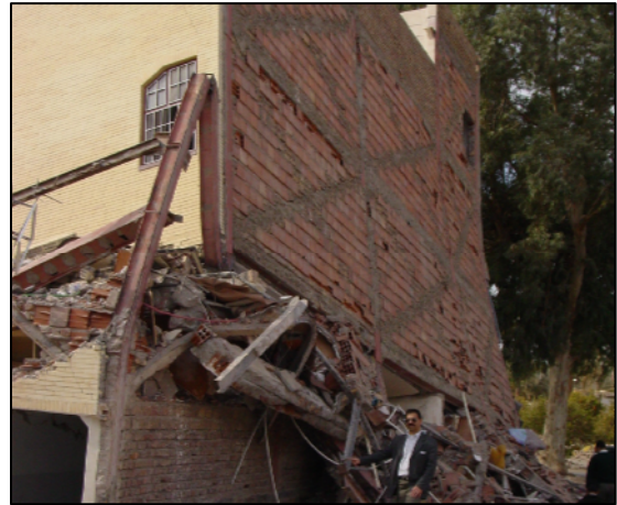
Figure 3 North view of building ST1 and failure of bracing connections
