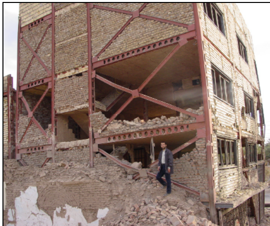
Figure 4 North view of building ST2 and failure of bracing connections
