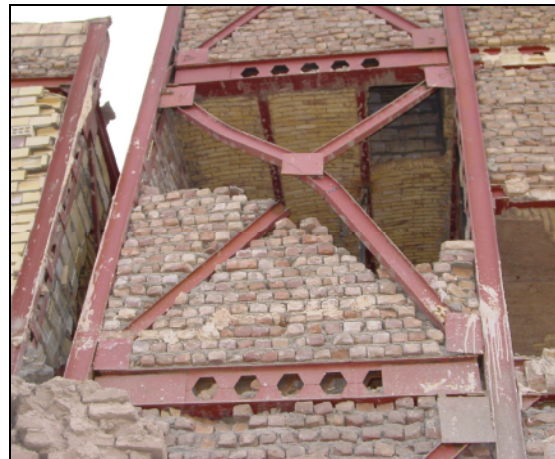
Figure 4 North view of building ST2 and failure of bracing connections
