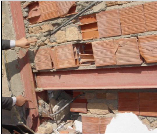
Figure 3 North view of building ST1 and failure of bracing connections
