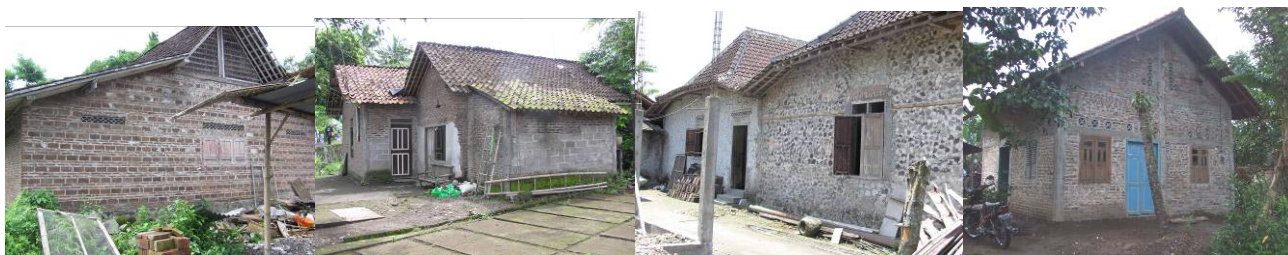
Figure 6 Non-engineered ordinary houses in Indonesia.
