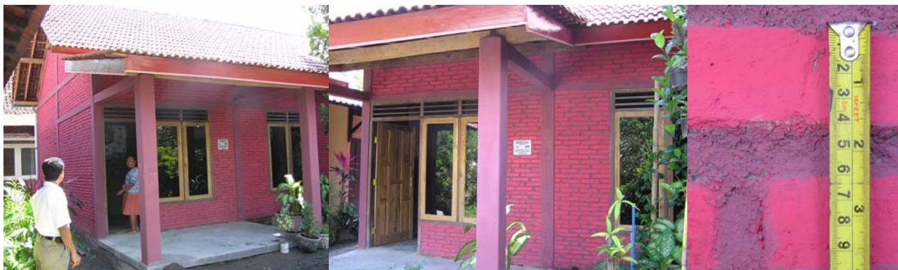
Figure 10. BARRATAGA model houses with adequate structural components and proper brick layering.
