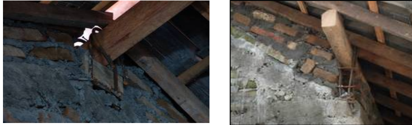
Figure 3. Column reinforcement hooked to the timber ridge and rafter
