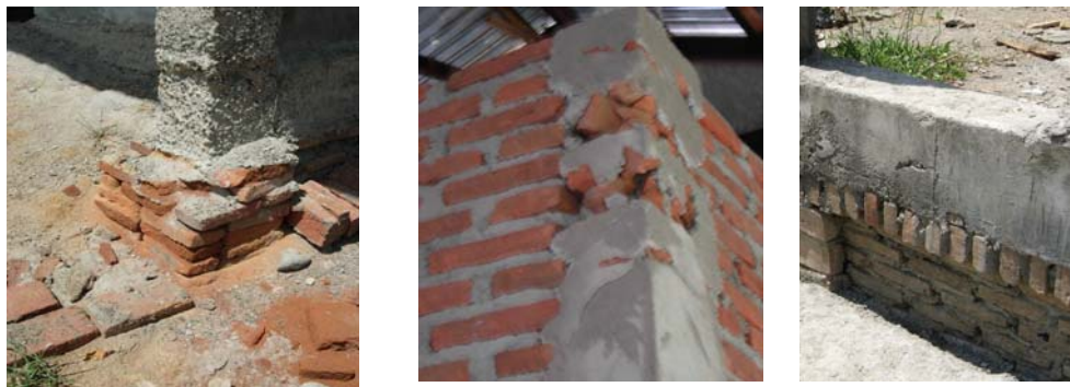
Figure 6. Brick for foundation, as concrete aggregate and for retaining wall
