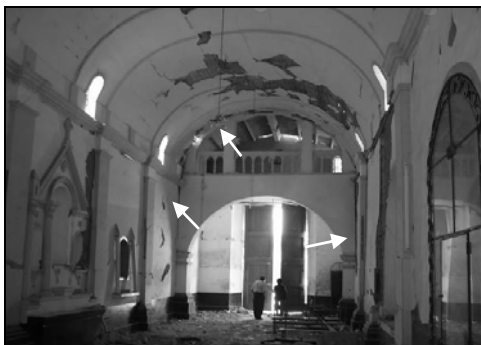
c) Detachment of the choir from the vault
