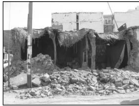
b) Eucalyptus trunks used as columns
