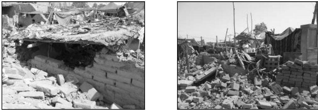
Figure 8 Collapse of buildings located on developing urban areas.
