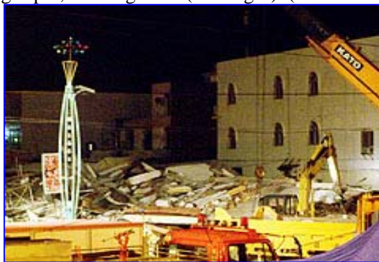
Fig.5 Zhengxing furniture shop collapsed
