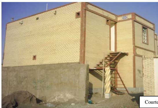
Figure 5 Connection of steel stairs to brick wall
