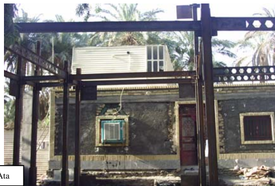
Figure 6 Use of castellated beams as main girders
