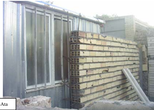
Figure 4 Using a container as a part of the house
