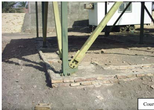
Figure 3 Use of bolt connections in steel frames
