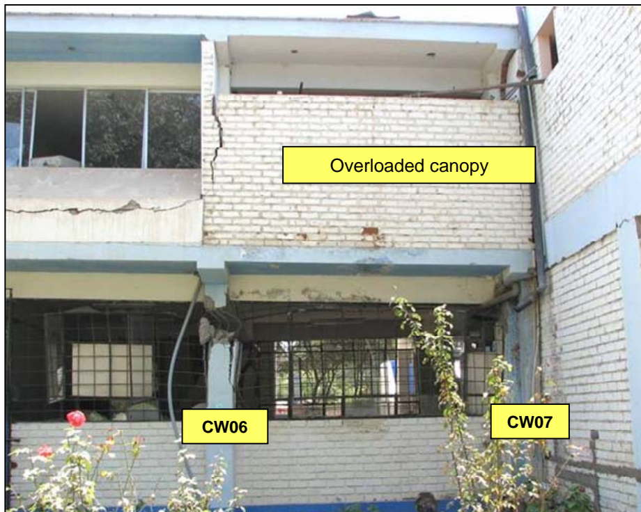
(c) Overloads from infill walls and canopy
