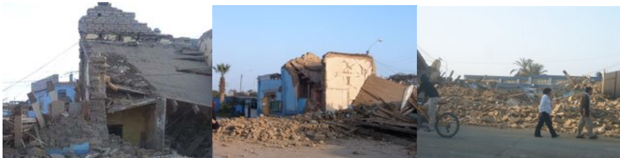
Figure 2: View of adobe buildings collapsed
