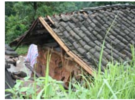
Fig. 9 Phenomenon of tile-slipping
