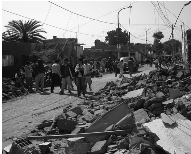
Figure 7 Non-engineered structures in Pisco, Peru 2007 Earthquake
