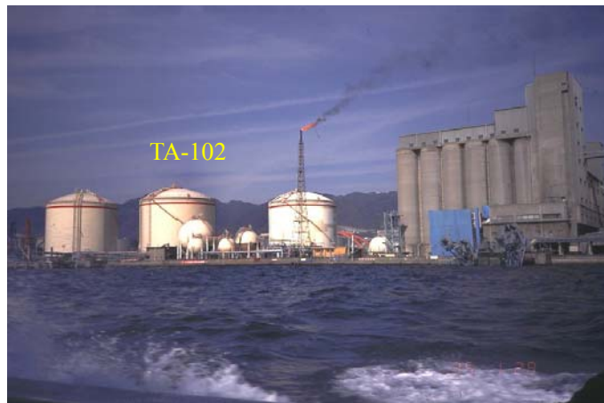
Photo 1 Damage to tanks during the 1995 Kobe earthquake
