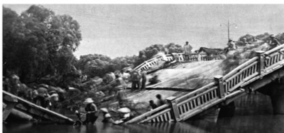
Figure 3 The destructive Shengli Bridge
