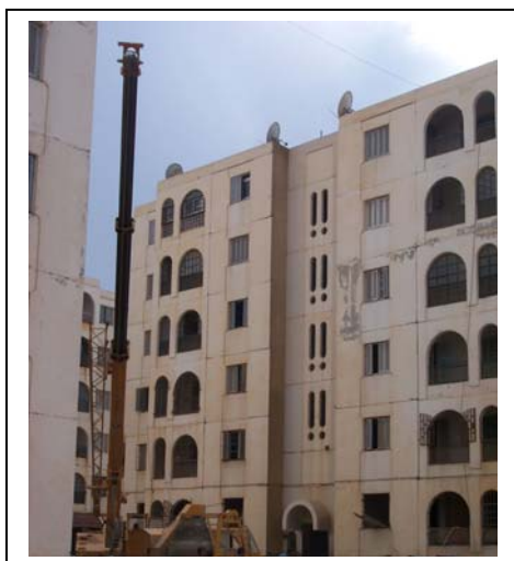
Photo N° 01: front view of the building
