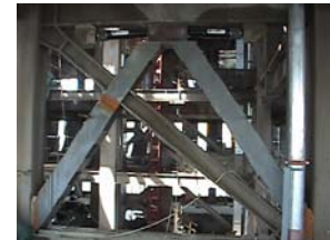
Fig.8 Cross Brace Damper
