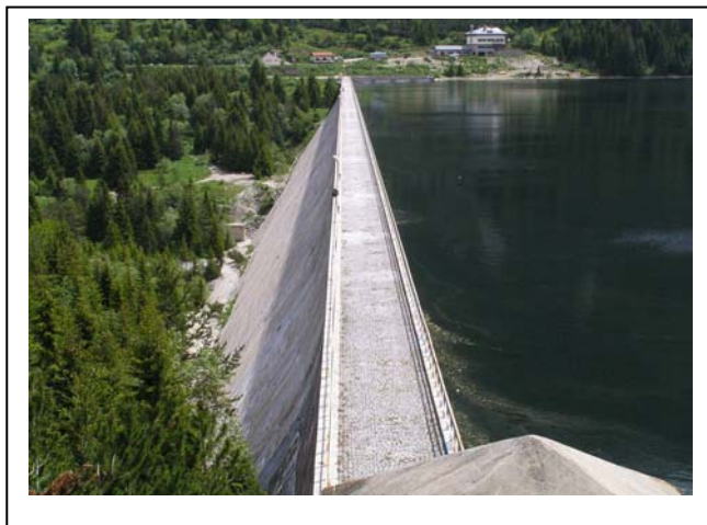
Figure 1. DAM 1 – global view
