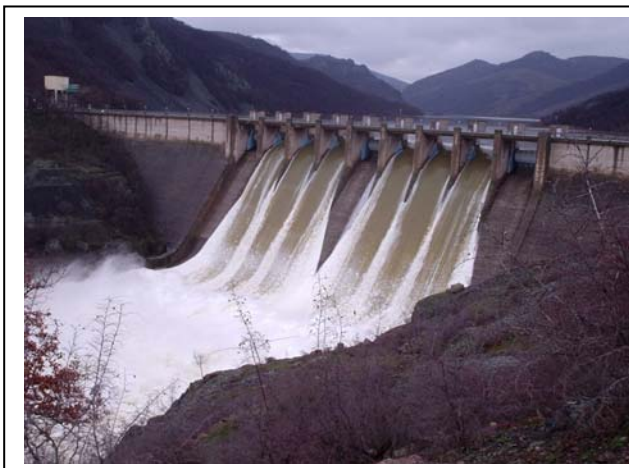
Figure 3. DAM 2 – global view
