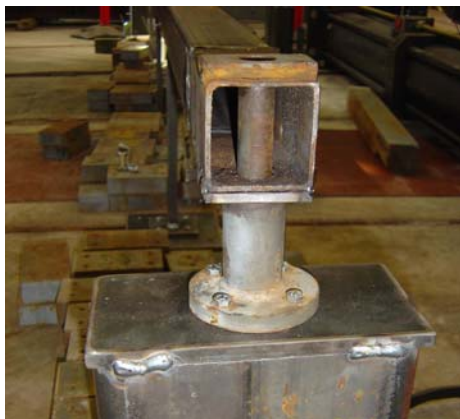
Figure 5. Abutment pin connection.
