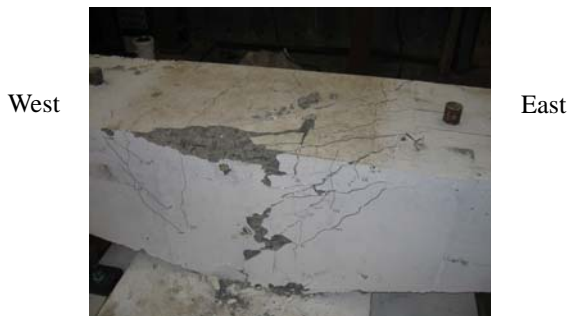
Figure 5 Damage in the regular beam
