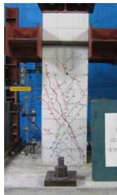
Figure 4.2 Crack patterns at the maximum strength
